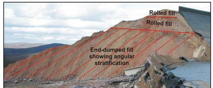
Fig. 2. – North side of the breached embankment shows the lower three quarters was end-dumped while the upper quarter was placed into two sequences of rolled filling. There does not appear to have been any significant effort made to mechanically compact the embankment because it was assumed to be a clean rockfill.
